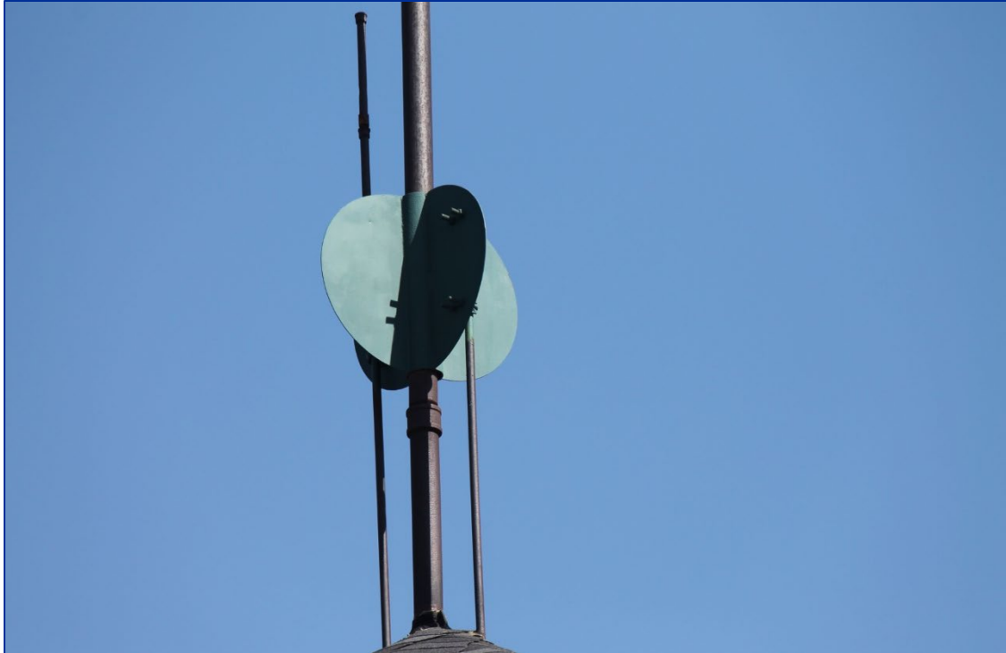
Photo 7: View of the metal float rod on the rooftop.
