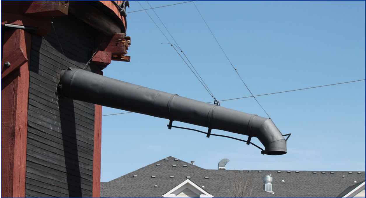
Photo 12: View of the metal spout.
