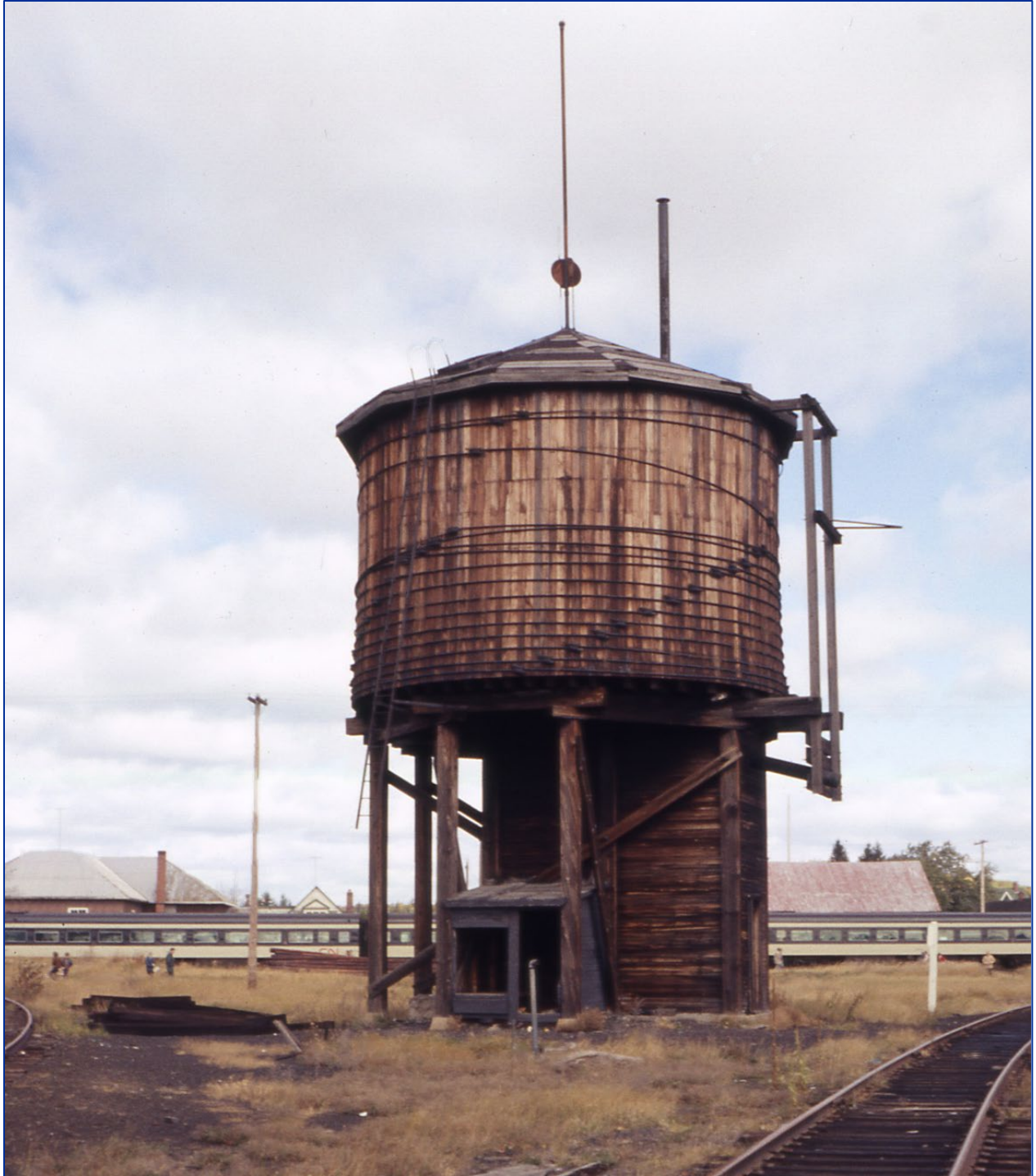
Image 8: View of the Water Tower with a small lean-to shed structure, 1972. 63
