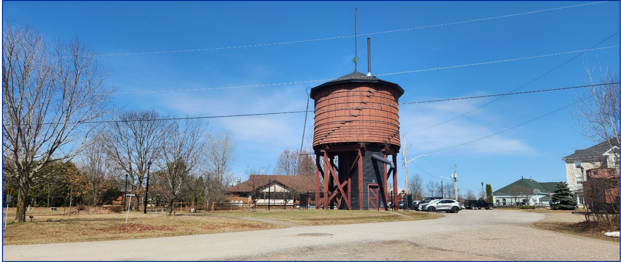
Photo 2: View along Mahon Street looking west towards the Water Tower.
